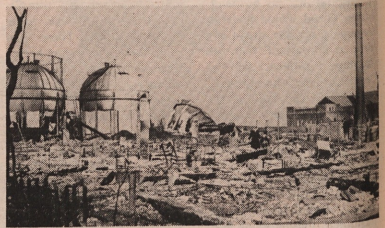
The two ball liquid gas storage tanks at left remain intact while the third one exploded when the cylindrical tank fell on it.
