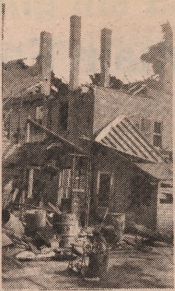
Little remains of a fire-gutted home on E. 61 St. after the spectacular explosion.
