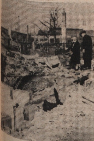
People search through the rubble that once was their home and sadly discover that everything they cherished is suddenly gone.
