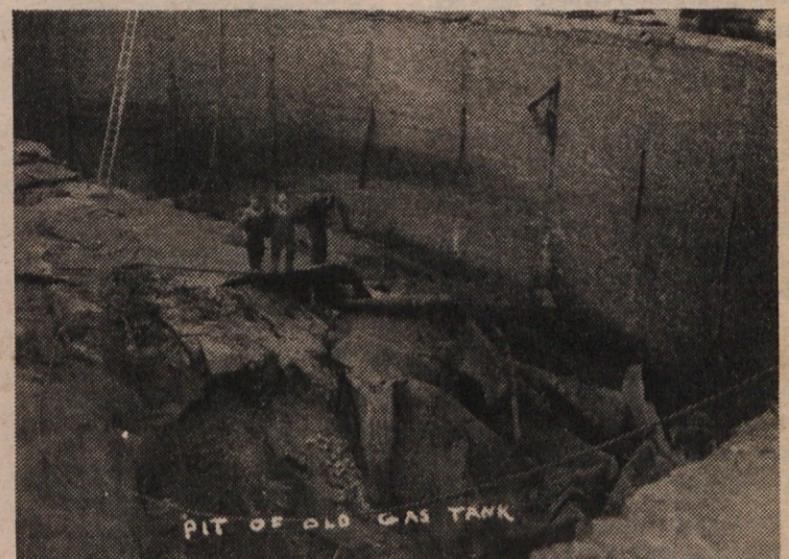
The three workers help demonstrate the tremendous size of the foundation of a gas tank which exploded.
