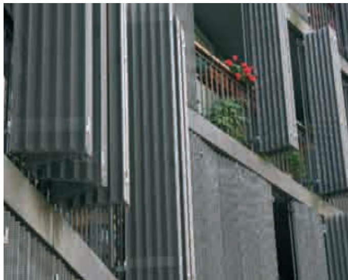
Slika 11: Zložljivi kovinski paneli iz kovinske mreže na ulični fasadi večstanovanjske zgradbe na Rue de Suisse (Herzog & de Meuron, Paris, 2000) [ http://housingprototypes.org/project?File_No=FRA023 ]. Figure 11: Folding metal net panel on the frontage of a multi-dwelling residential building in Rue de Suisse (Herzog & de Meuron, Paris, 2000) [ http://housingprototypes.org/project?File_No=FRA023 ].
