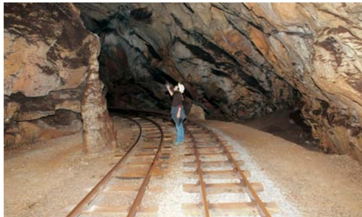
*Fig. 5: The cave railway in Postojnska jama: the embankment covers the whole of the passage. The rust particles are raised into the air by the draught and settle on speleothems and rock. Part of the embankment where the gravel has been replaced is still white.*
