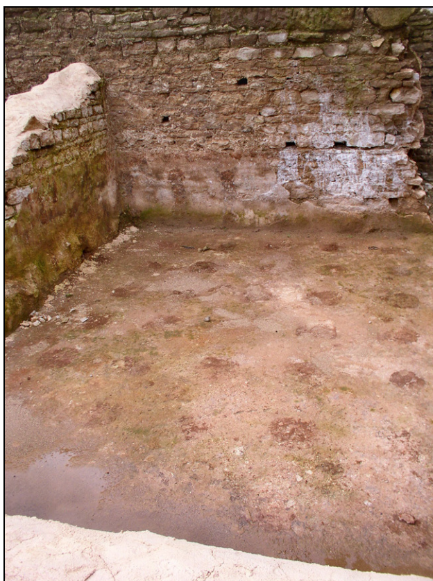
Fig. 24: Floor of caldarium (P1-O4) with traces of pillars (photo: A. Starac). Sl. 24: Tla caldariuma (P1-O4) s sledovi stebrov (foto: A. Starac).
