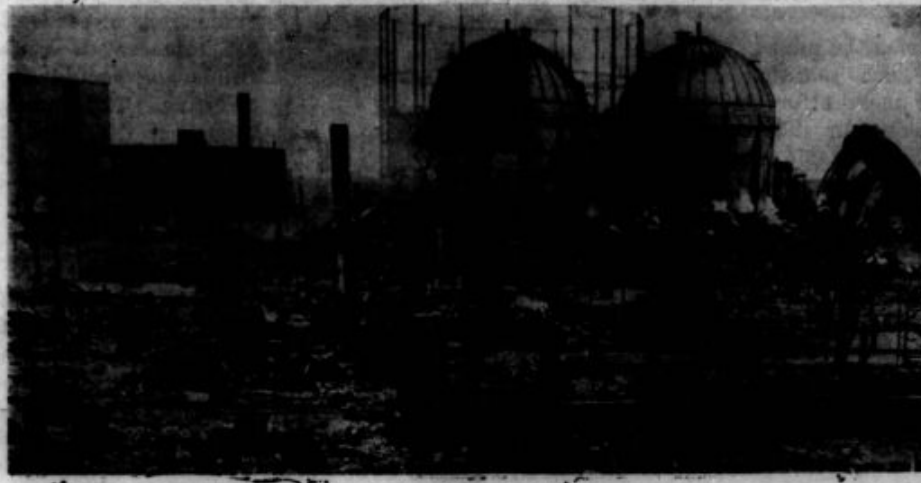
This is part of the scene of devastation caused by explosion of a liquid gas storage tank of the East Ohio Gas Co. Looking north from E. 61st St., two tanks which magically escaped destruction are seen above the rubble of wrecked homes.
