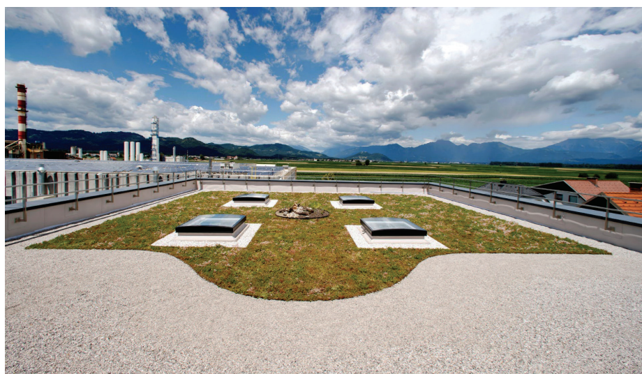
Slika 2 • Knauf Insulation Experience Center – zelena streha.
