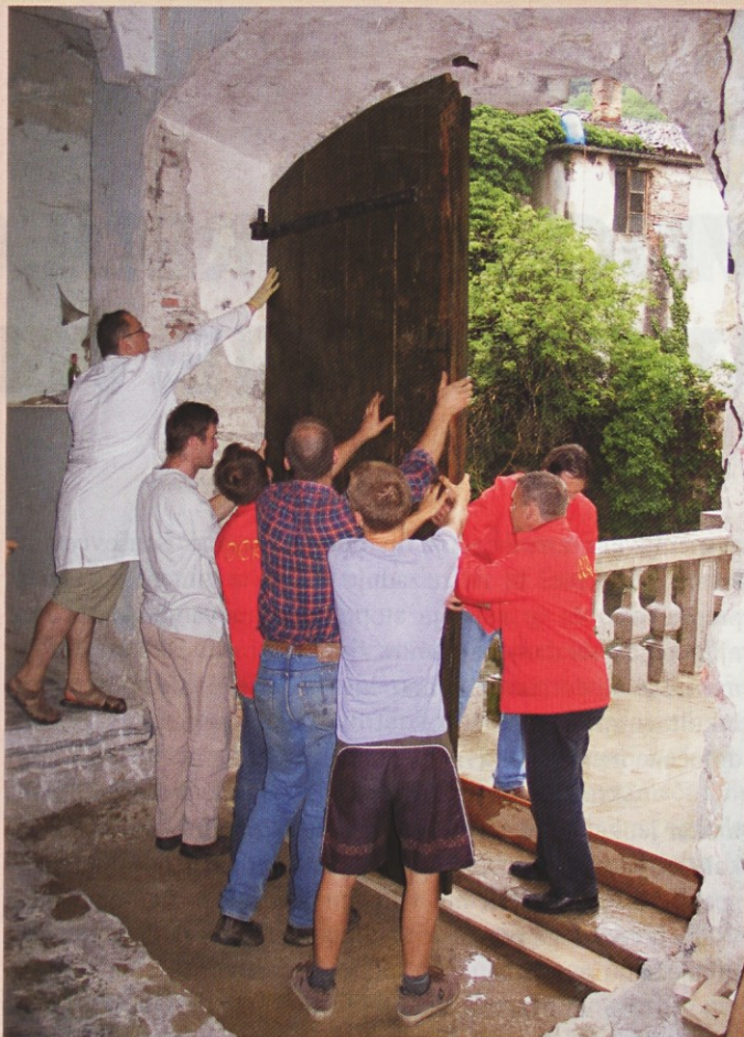
Delavnica mizar, restavratorski sodelavec: montaža vrat
