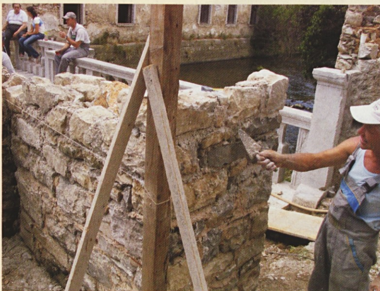
Delavnica zidar, restavratorski sodelavec: zidanje kamnitega zidu
