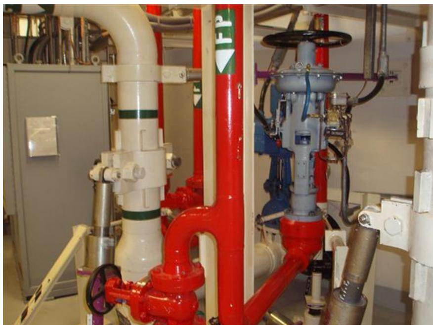
**Figure 12: Fire insulation valve 28985 (the valve is located on the fire pipe for extinguishing reactor coolant pump No. 1)**
