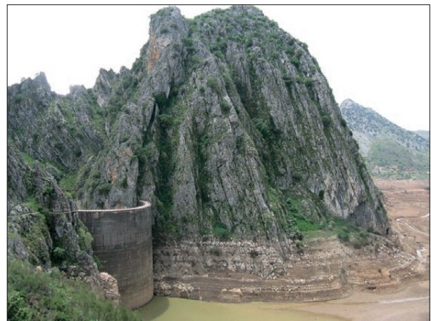
Fig. 12: Empty reservoir of Montejaque dam on Gaduares River in karst of southern Spain. Due to high leakage the reservoir was abandoned in the 1950s (Photo: Z. Stevanović).
