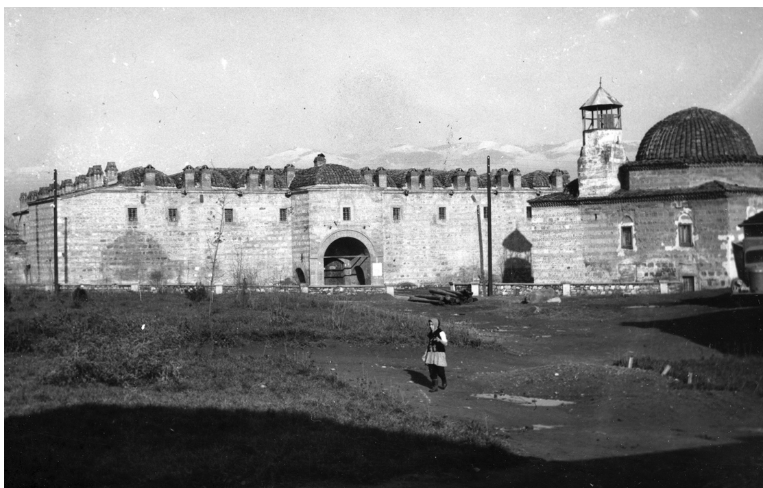
Fig. 153 Museum of South Serbia in Skopje in Kurshumli an building (early 1920s). Courtesy of the Archaeological Museum of Republic of North Macedonia.
