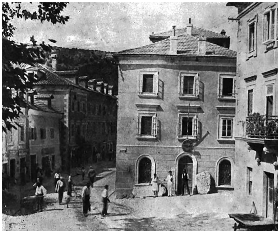
Fig. 66 Fontana House in Knin, venues of the Museum of Croatian Antiquities between 1893 and 1934 (Gunjača 1958).
