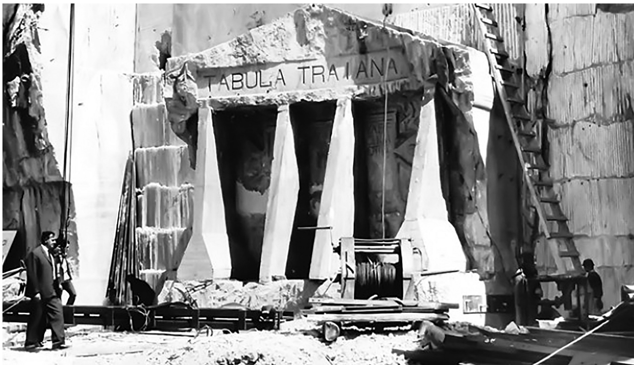
Fig. 103 Relocation of Tabula Traiana (1967–1969) during the construction of the Đerdap powerplant. Photo Mihailović M. (2016).
