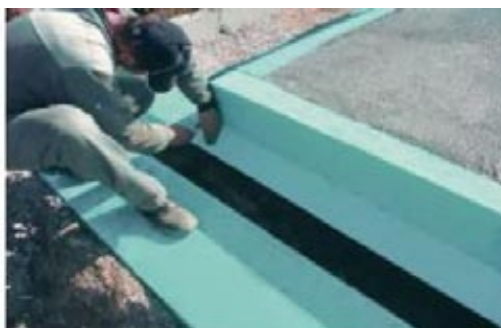
Figure 6: Placing of XEPS isolation
