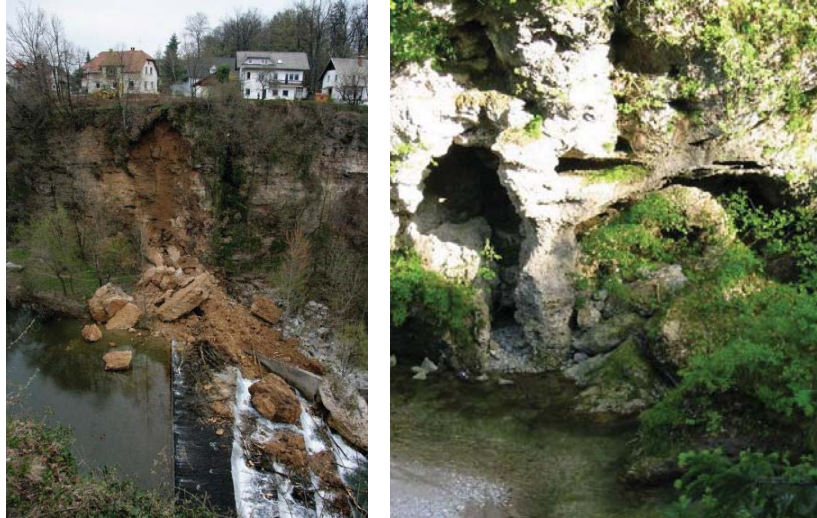
Several caves of the old Carniolan conglomerate Karst, which still collapse 105 [pic.241,242] – the rockfall on 4 November 2010, when over 100 cubic metres of conglomerate walls crashed
