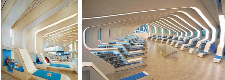
Glued laminated timber structures GLTS - Vennesla Library and Cultural Centre by Helen & Hard Architects [pic.223, 224]
