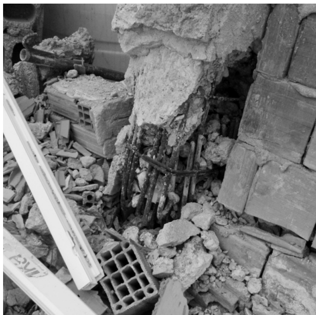
Figure 1: Corrosion of the reinforcement in a damaged column observed after the Van earthquake of 23 October 2011 (Murat Öztürk's archive)
