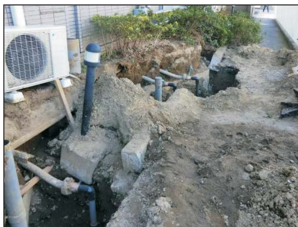
Figure 17. Settlements of the ground around buildings with deep foundations in Katori city.
