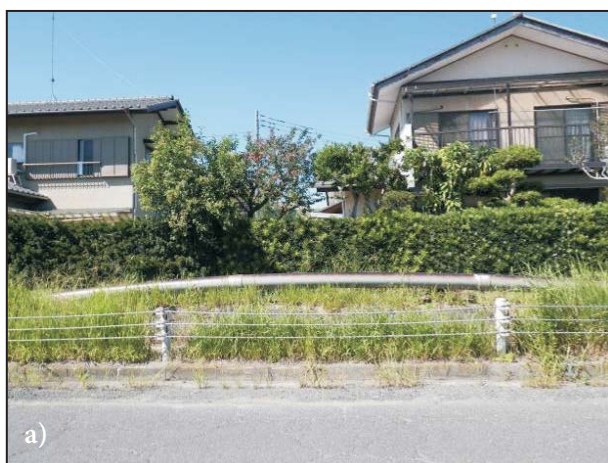
Figure 15. Uplift of (a) pipeline in reclaimed land of Itako city and (b) underground tank in Kozaki town.
