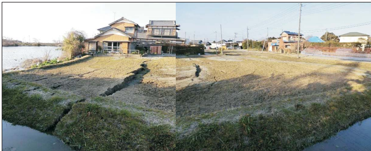
Figure 16. Lateral spreading with a maximum horizontal displacement of about 1 m in Katori city.
