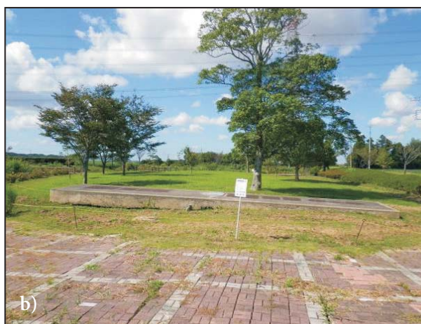
Figure 15. Uplift of (a) pipeline in reclaimed land of Itako city and (b) underground tank in Kozaki town.
