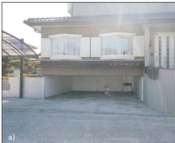
Figure 14. Residential houses in Itako city settled (a) evenly or (b) with tilting.
