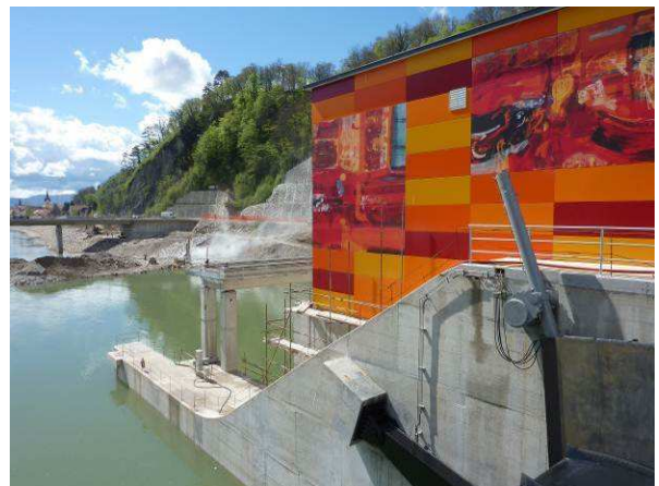
HE Krško – Fasada stronice in v ozadju novi most obvoznice Krško.
