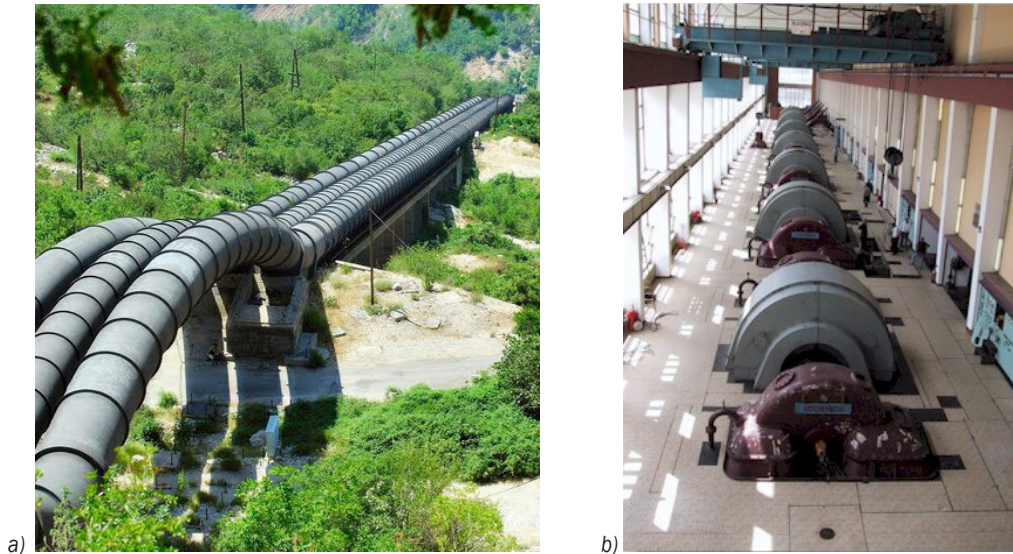
Fig. 3. Layout of a) three parallel penstocks and b) powerhouse with seven twin-type Pelton units in Perućica HPP
