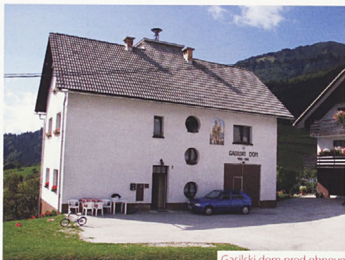
Gasilski dom pred obnovo
