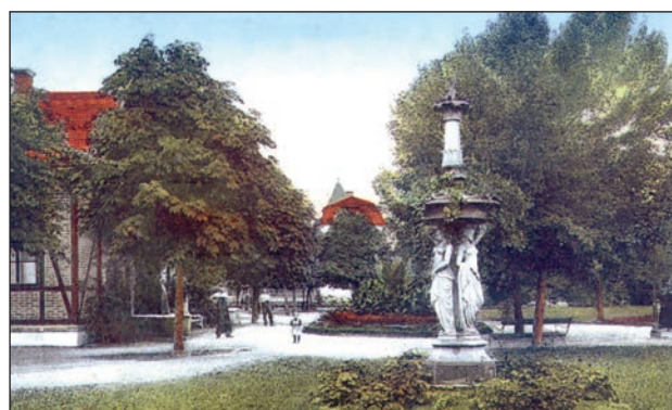
Fig. 10. Karlovac, Vrbanić Park, early 20 th century, source: private collection
