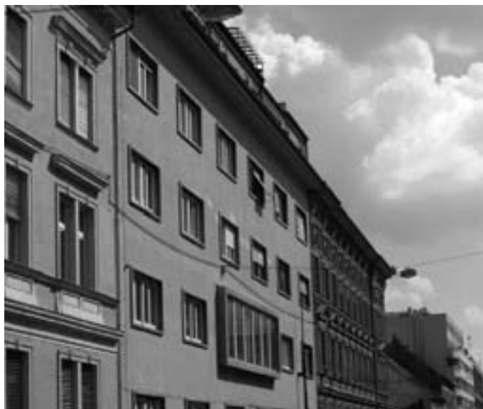
Slika 6: Večstanovanjski blok. Figure 6: Apartment block.
