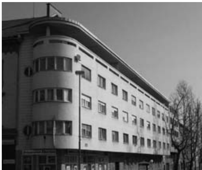
Slika 5: Večstanovanjski blok. Figure 5: Apartment block.
