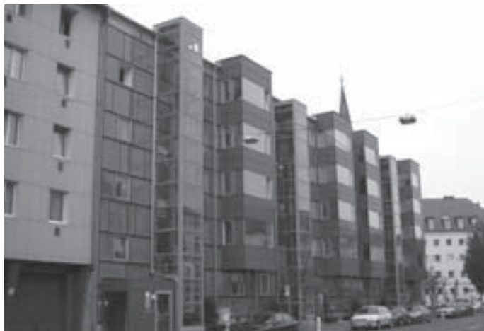
Slika 11: Sanacija večstanovanjskega objekta v pasivnega, Linz, Avstrija. Figure 11: Remediation of a multi-occupied building and conversion into a passive one, Linz, Austria.
