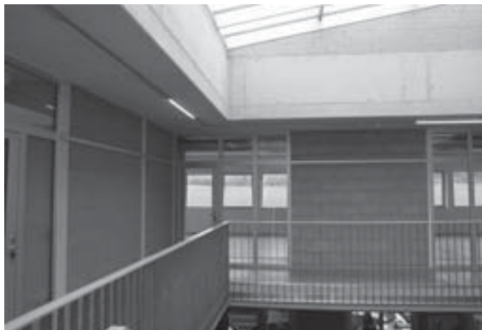
Slika 6: Stene iz nežganih ilovnatih zidakov shranjujejo toploto. Figure 6: Walls of unfired clay bricks keep warmth.
