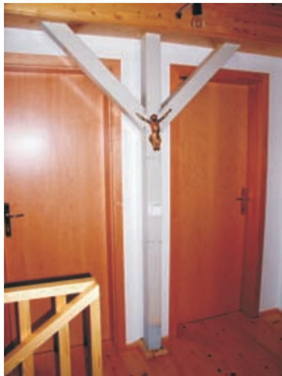
Slika 7: Nosilni steber strehe. The roof's load-bearing column.
