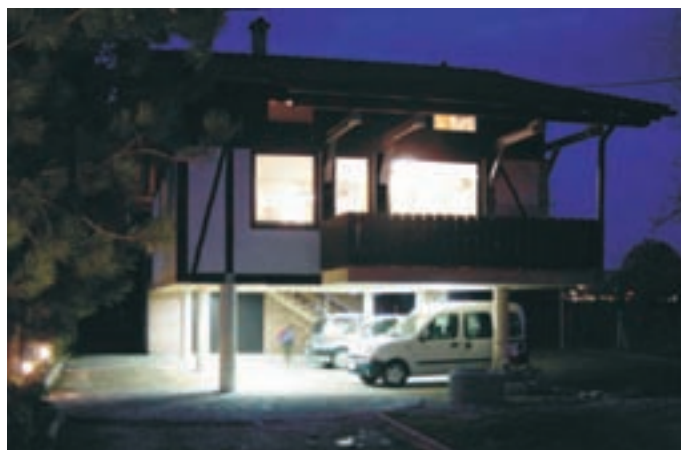
Slika 4: Pogled na objekt s ceste (ponoči). A view of the building from the street (night).
