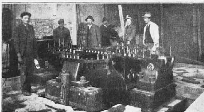
Sl. 6. Montiranje parne turbine
