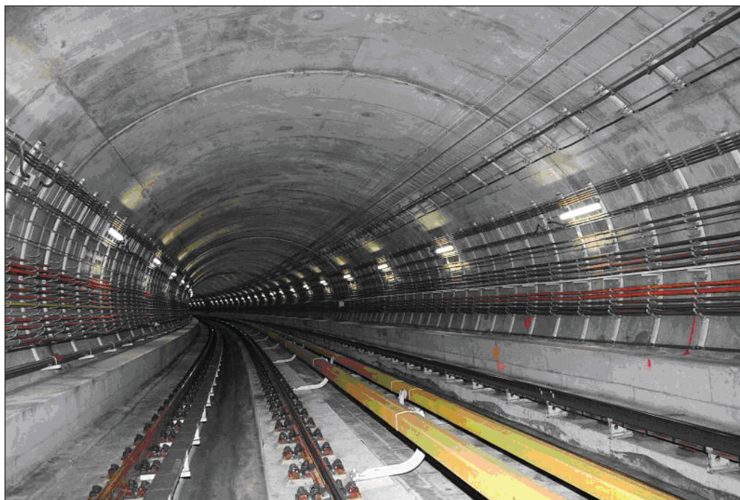
Figure 3. Double-track metro tunnel on line C.
