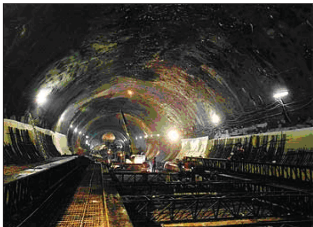
Figure 8. The building of the Kobylisy station.
