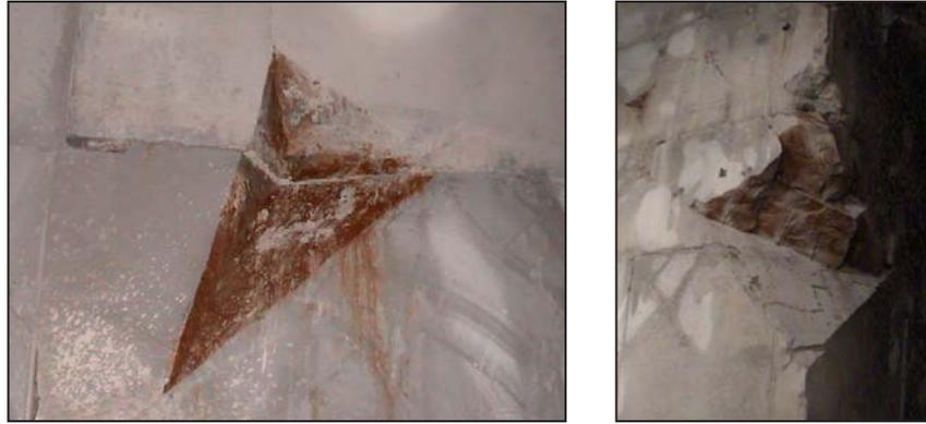
Figure 4. Samples of falling rock wedges in underground structures of Lipica II. quarry.
