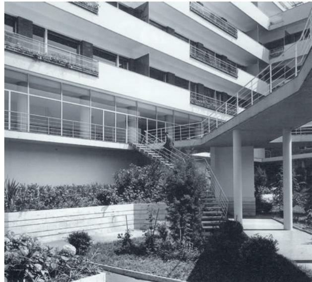
that the first project of a steel construction tower with many windows overlooking a small square, was replaced by a structure in reinforced concrete leaning on a large basement. There is an interesting top floor with a restaurant with glass curtain walls, that was in the original design. Unfortunately this project was strongly criticized for political reasons.
