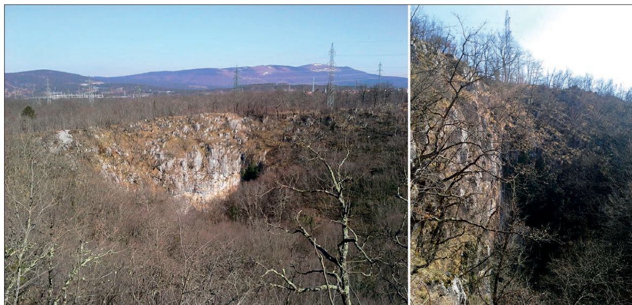
Fig. 5: Frontal (right) and lateral (left; towards the SE) view of the cliff originating along the Risnik Fault plane in the Bukovnik collapse doline.
