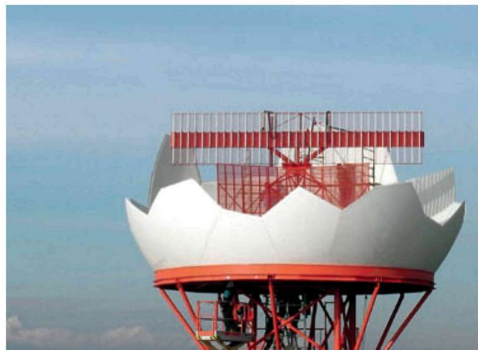
A radome protects two antennae of PSR and MODE-S radar at Jože Pučnik Airport.
