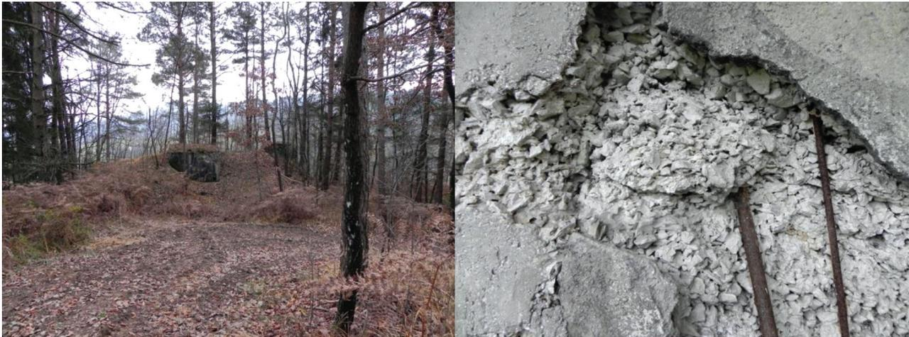
**Figure 1:** Ridgetop bunker perfectly blended with nature (left) and poor concrete compaction due to low workability (right)
