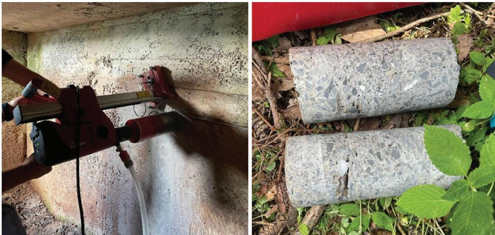
**Figure 3:** Coring of the concrete samples (left) and concrete cores taken from the lowland bunker (right)
