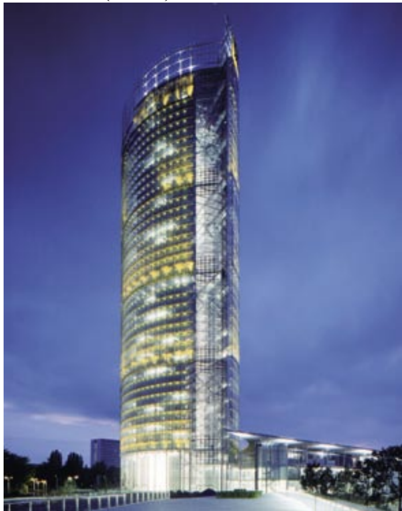
Post-Tower v Bonnu (162 metrov).
