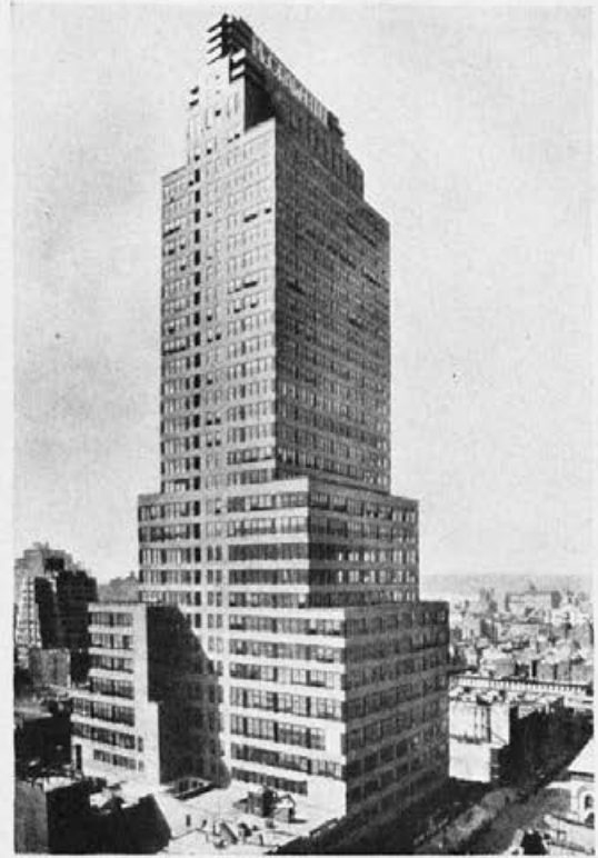
Mac Graw-Hill-Building, New York (1931)
