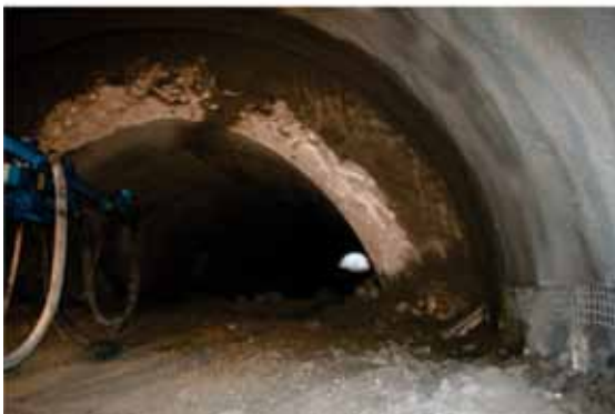
Figure 8. The final cross-section of right tunnel tube after reconstruction.
