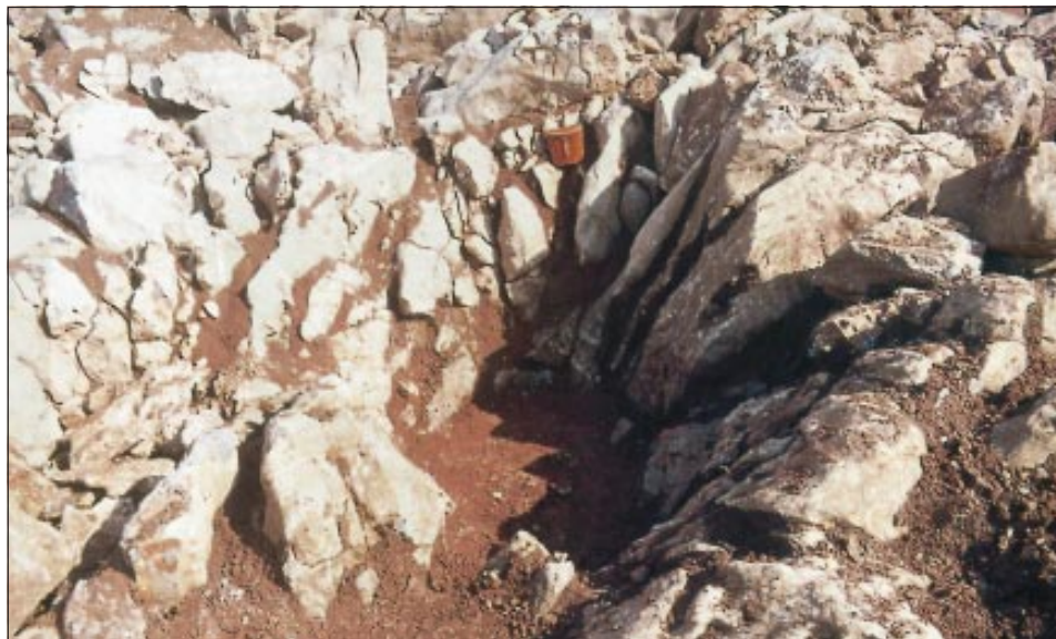
Photo 1: Subsoil doline with stripped off soil in the quarry at Podutik. The main crushed zone is crossing the less effective one in the middle of the doline.
