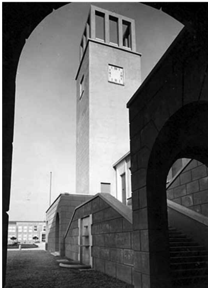
Fig. 7: Piazza del Municipio (Town Hall Square). Design and current state (Association "Primi di Torviscosa" historical photographic archive, there).
