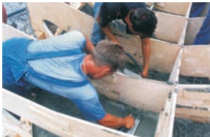
Slika 15: Zgornji profili in betoniranje lupine. (foto: Marmor Hotavlje) The upper profiles and concreting of the shell.
