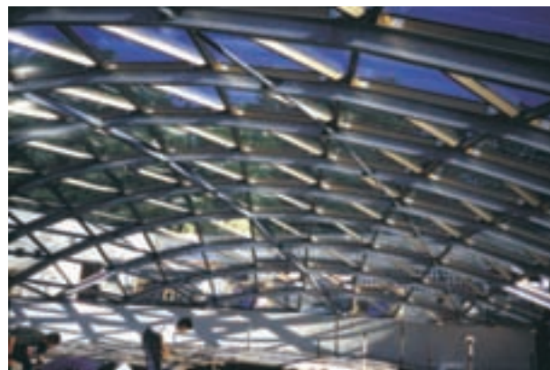
Slika 4: Dejanska montaža lupine. (foto: Aluterm) The actual assembly of the shell.
