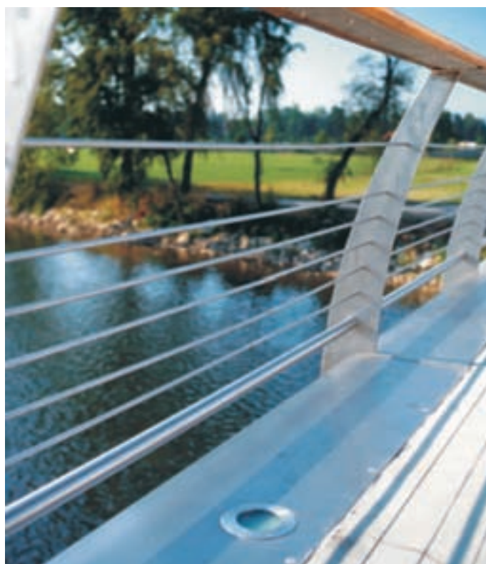
Slika 7: Mostna ograja ima široko mostno polico in niz svetilk, skritih v zaključnem vencu objekta. (foto Miran Kambič) The bridge parapet has a wide bridge shelf and rows of lights hidden in the bridge's concluding cornice.
