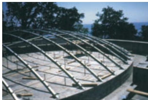
Slika 4: Dejanska montaža lupine. (foto: Aluterm) The actual assembly of the shell.
