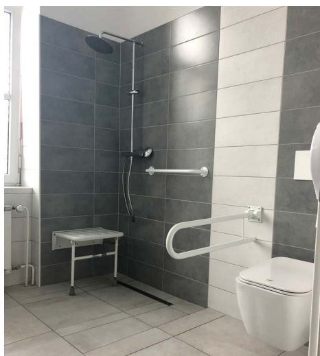
Figure 1: An example of renovated sanitary facilities in isolation rooms before the coronavirus epidemic
