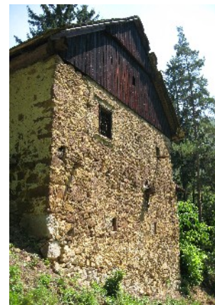
JZ stena prizidka
