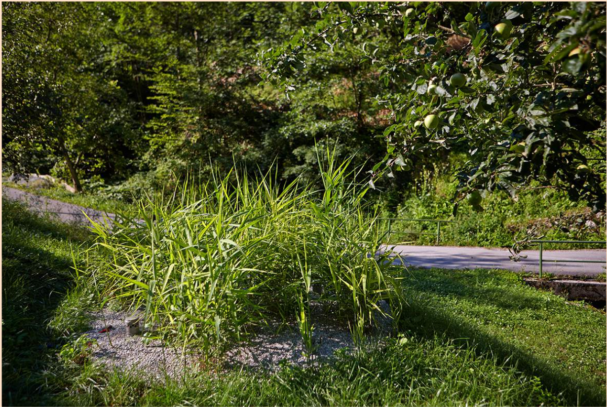
Figure 2: VFTW for wastewater treatment from single household with capacity of 4 PE. Photography taken by Iztok Ameršek.
