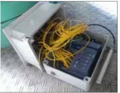
**Figure 5.** Operating console for the remote control of the mobile hydraulic platform
