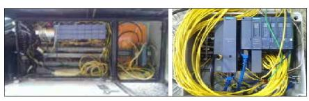
Figure 4. Main distribution cabinet after reconstruction procedure
