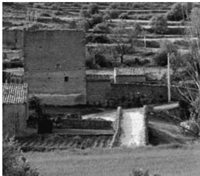
Figure 2: The intervention recently carried out in the bridge of Pobleta de San Miguel in Villafranca del Cid (Castellón) was aimed at the restoration of the medieval monument and the recovery and valuation of its surroundings.
