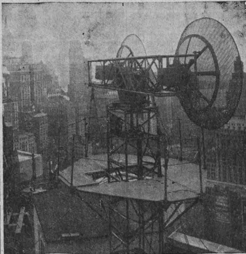
Shown atop the New York telephone building are the antennas used during demonstration of a secret army radar microwave relay system. The demonstration, conducted by Bell telephone laboratories, included a two-way voice transmission carried out successfully over links totaling 1,400 miles. It was announced as entirely practical and successful.
