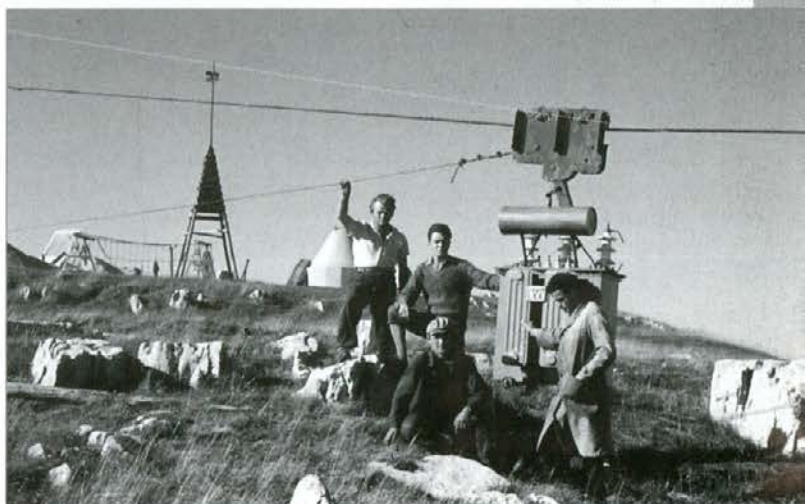
Transformator na 1696 m
