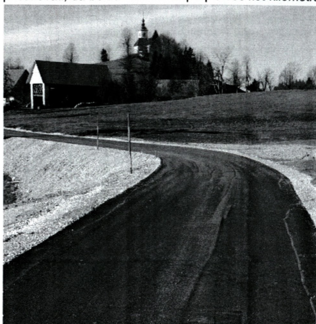
Nov asfalt in urejene bankine (foto R. B.)
