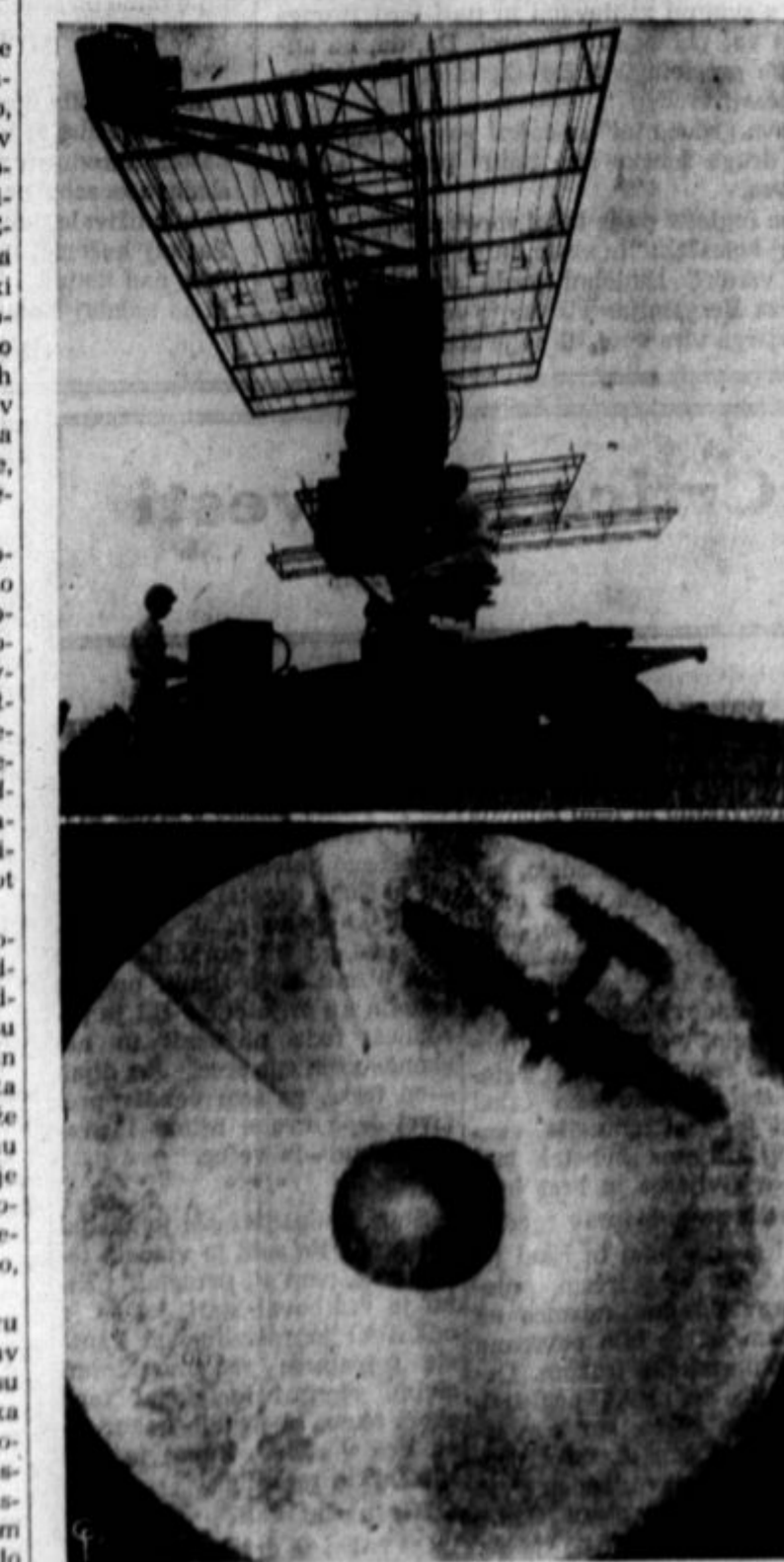
SOLDIERS OPERATE a mobile-trailer mounted radar set (top) during a demonstration in which the secret surrounding the device was lifted. This particular type of machine was attached to searchlights and anti-aircraft guns and automatically gave the range of enemy aircraft that came within its beam. At bottom, the image of a low-flying bomber is picked up on the illuminated oscilloscope the moment it comes within range of the machine and, almost immediately after the plane's shadow appears, ack-ack guns begin to fire at it. A. A. F. Photos.
