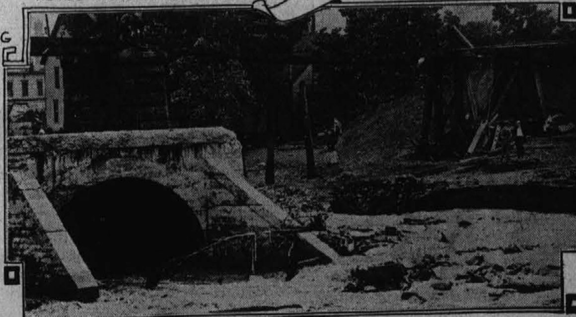
WRECKED NICKEL PLATE BRIDGE AT 19TH ST.
