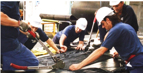
Fig. 2. Preparation process of a steel cord splice [RI-Belt Sud S.R.L.]
