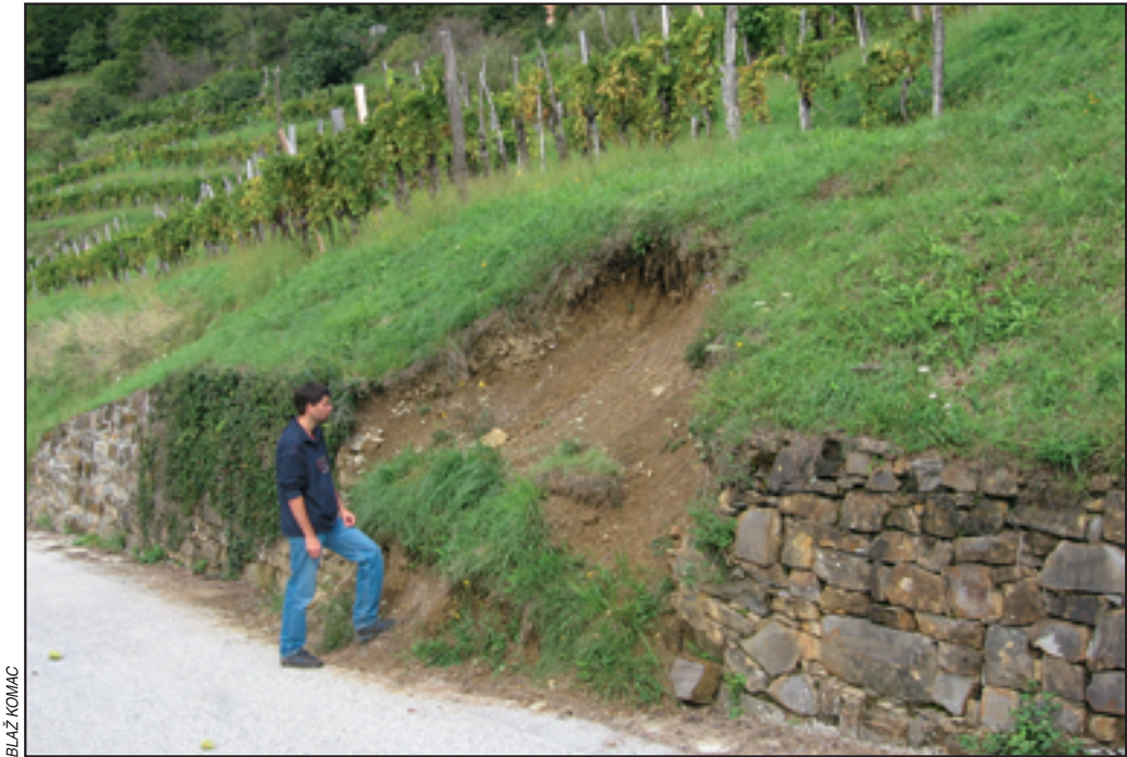
Figure 4: Stone walls collapse when they can no longer hold back the landslide.
