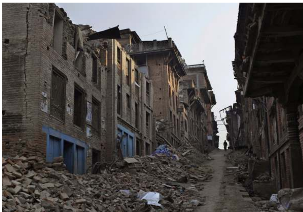
Slika 4. Poškodovane hiše v Katmanduju. Vir: http://www.theatlantic.com/photo/2015/07/nepal-three-months-after-the-earthquakes/399773/
