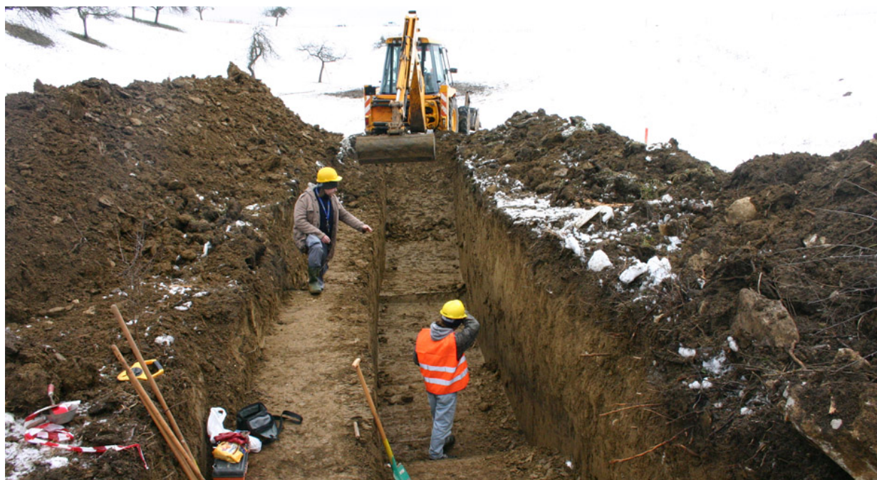
Figure 13 Machine excavation of test trenches (archive IPCH, CPA).
