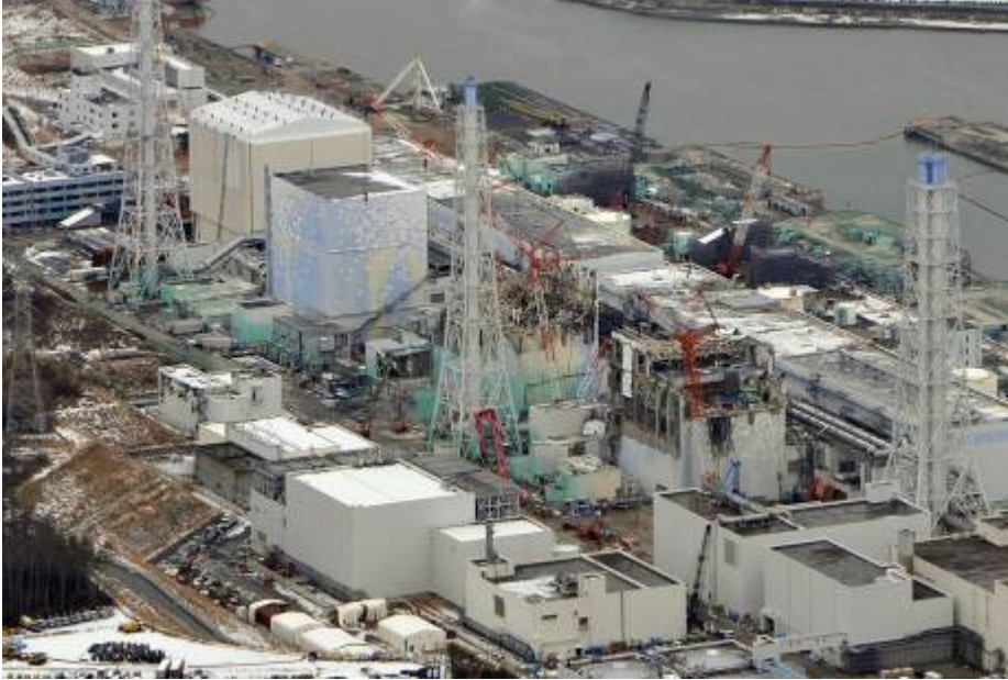
Figure 21: Fukushima I NPP after the earthquake
