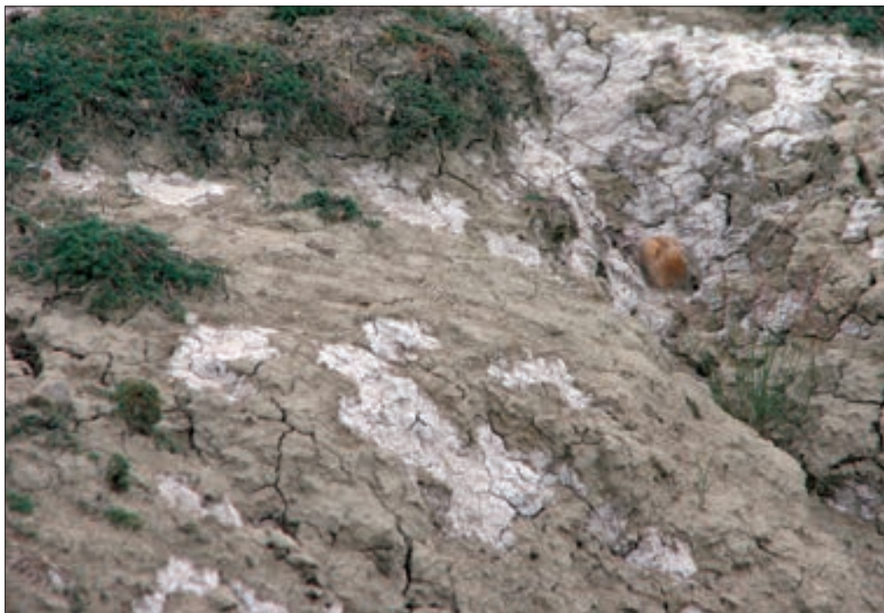
Thin layer of salt is accumulated on flat and gently sloping surfaces.
